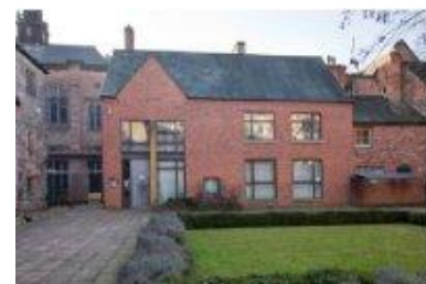
Our New Offices at Castle Yard
